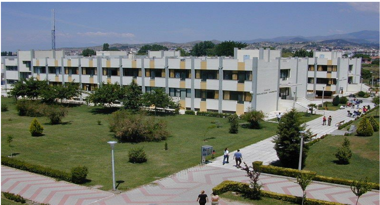
View of the Department's main building
